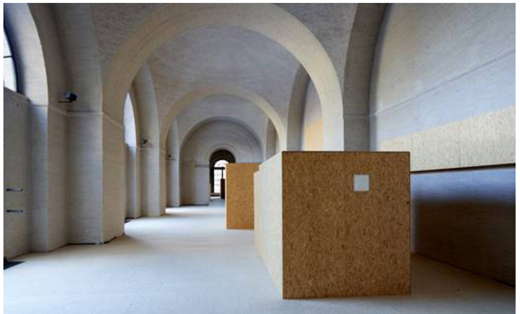
Fig. 1: Covered floors and enclosed sculptures in the Roman Hall. (Photo: St. Müller-Naumann)
