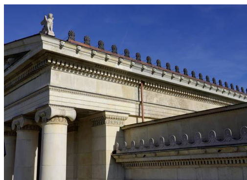
Fig. 2: Restored architectural ornamentation. (Photo: M. Pfanner)
